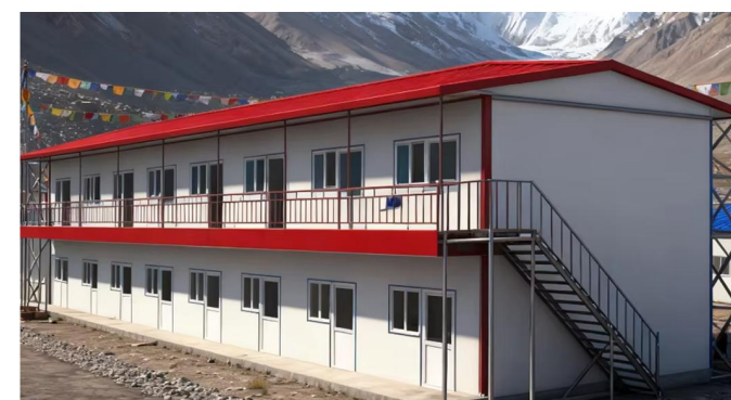
Public utilities room
