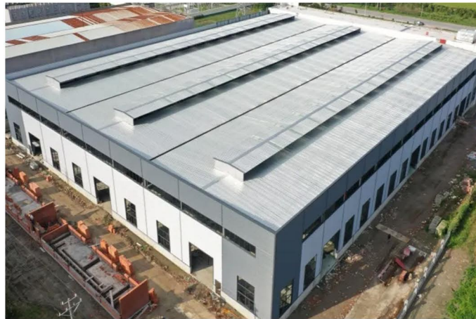
Steel structure building
